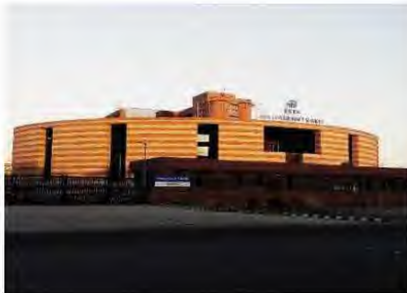
TCS Garima Park, Ahmedabad: LEED Gold Certified
